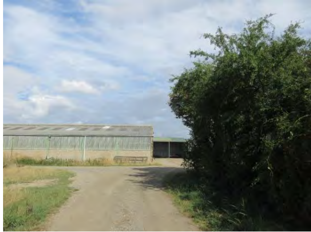
Photograph 16. Farm access through outbuildings. Load approaches camera. Negotiable with caution and with courtyard kept free of vehicles and any other items that could be in store.
